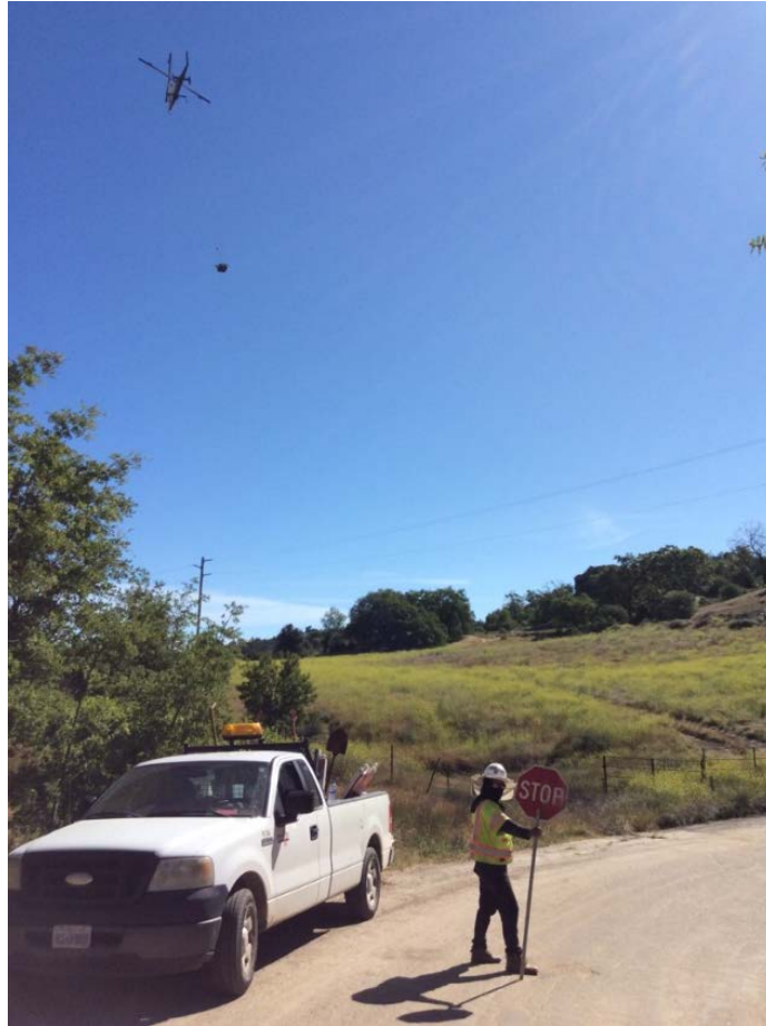
Photo 6: During helicopter external loads crossing Eagle Peak Road (TL 626 Conversion North (C 222)), traffic control measures were observed being implemented in accordance with the Traffic Control Plan (APM TRANS-05) and the ASP (MM PHS-5).
